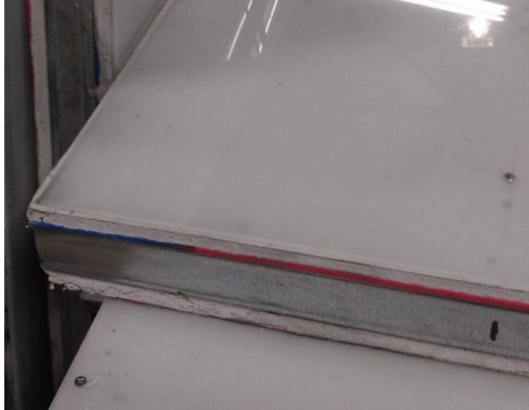
Figure 7-2. Thermoplastic three wall panels screwed to 5/8-inch drywall sandwich with steel studs
