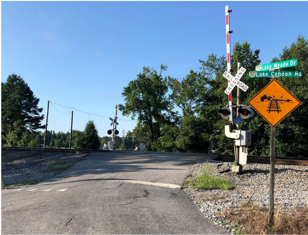
Figure 1 – Humped crossing in Suffolk, VA (Crossing ID 467411X)
