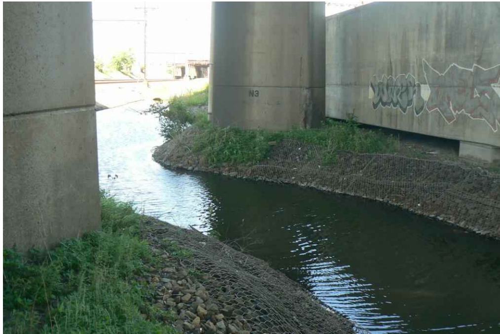
Open channel connection from Cedar Creek Marsh South. View looking west. Note gabion/rip rap shoreline.
