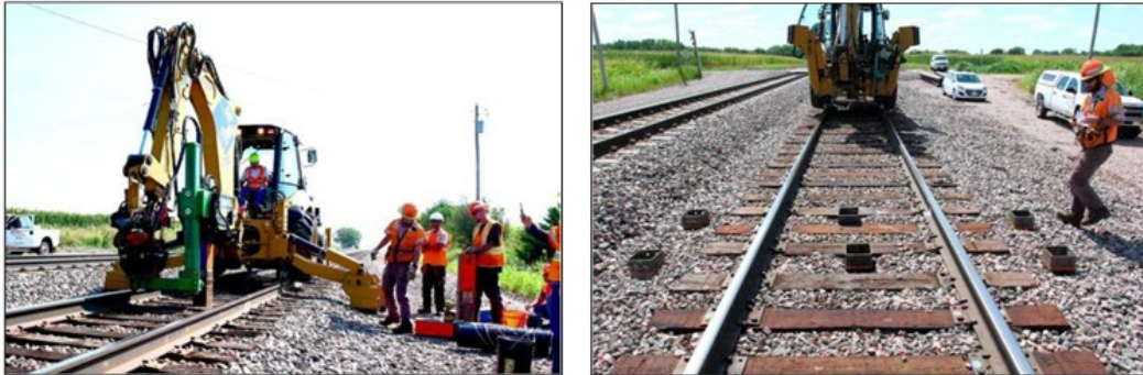
Figure E 3. (Left) BNSF TR&D vibro-sampler in operation at sample location #29. (Right) Emplaced sampling tubes at sampling location #22
