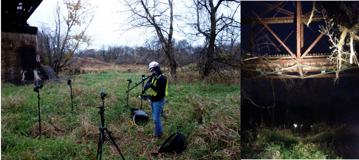
Figure 5.3 Camera and halogen lights in preliminary field test
