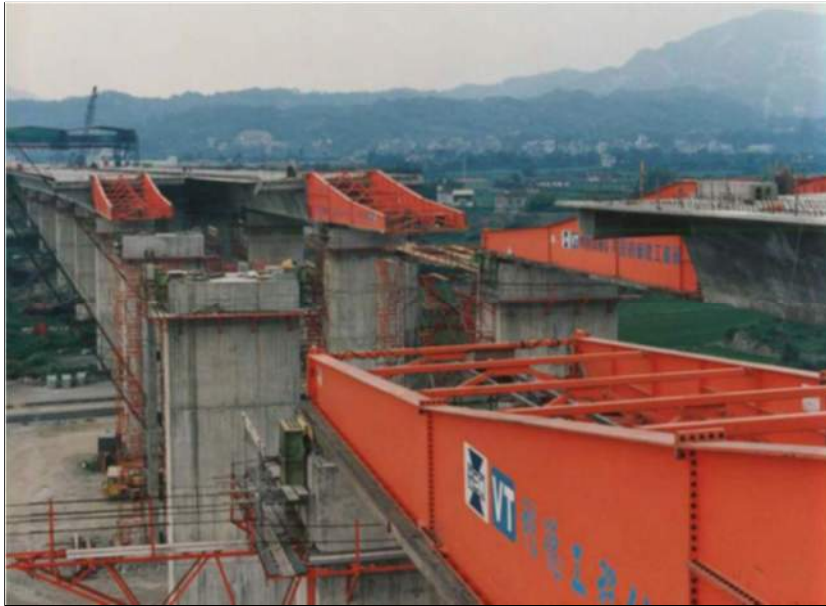
Figure 4: Incremental Launching Method Equipment Used on the Tou Chien Bridge Second Freeway, Taiwan (Photo courtesy of Wiecon)
