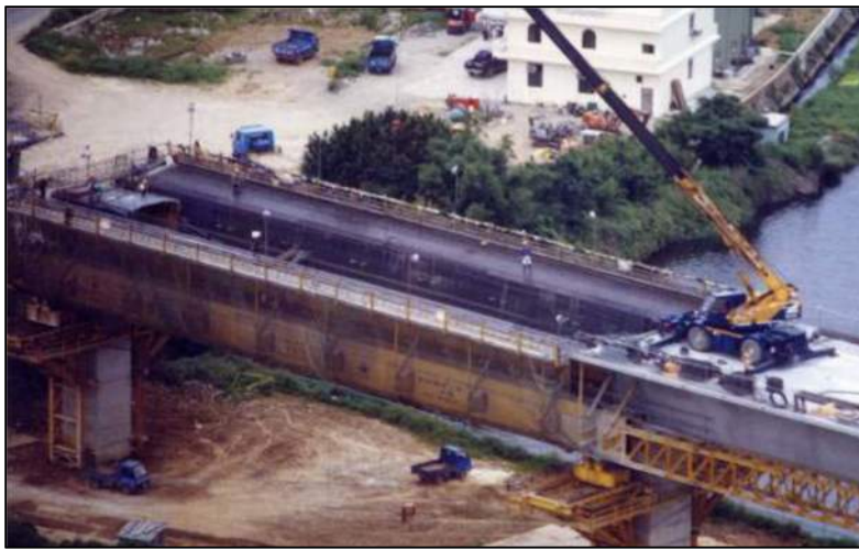
Figure 8: MSS in Place Awaiting in Situ Construction, Taiwan High-Speed Rail, ROC (Photo courtesy of THSRC)
