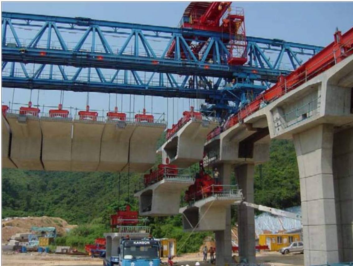
Figure 2: Deep Bay Link Bridge in Hong Kong, Precast Segmental Span-by-Span Method Using Overhead Gantry
