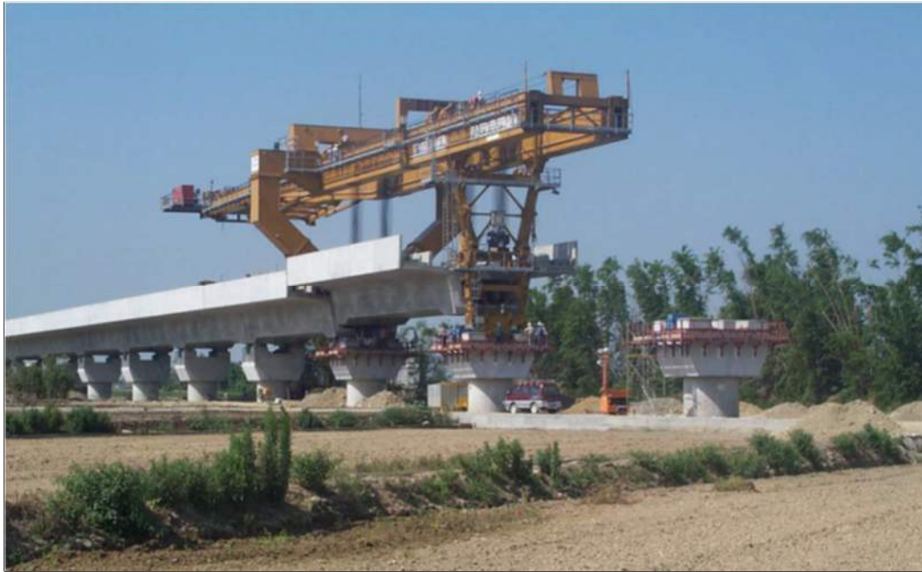
Figure 5: Launching/High-Speed Rail System under Construction in Taiwan, ROC (Photo courtesy of THSRC)
