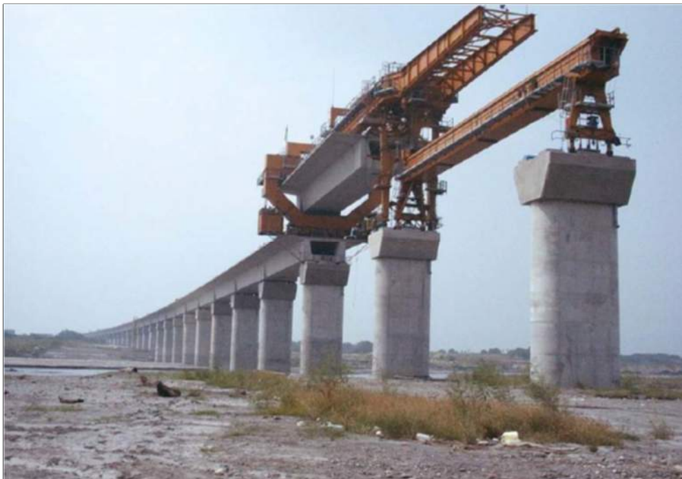
Figure 6: The Full-Span Precast Launching Method Launching/High-Speed Rail under Construction in Taiwan, ROC (Photo courtesy of THSRC)
