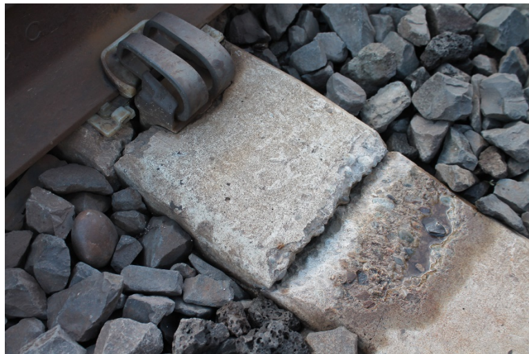
Crosstie Transversely Broken Between the Rail Seats
