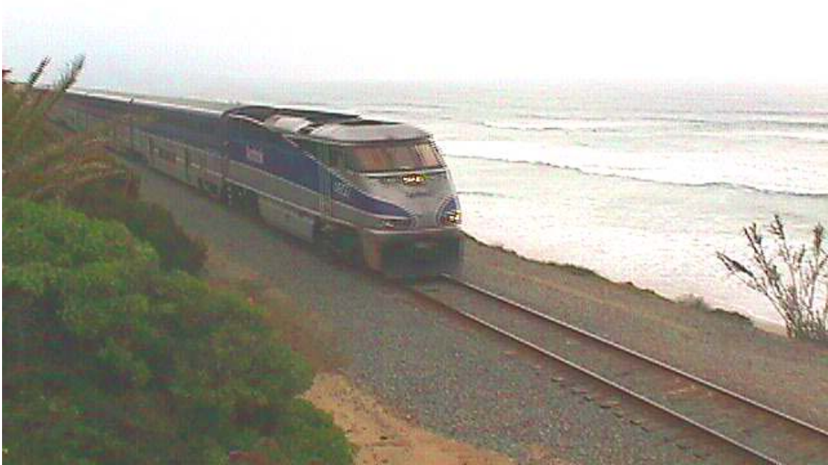
Figure 6-4 – Train passing along Del Mar Bluffs
