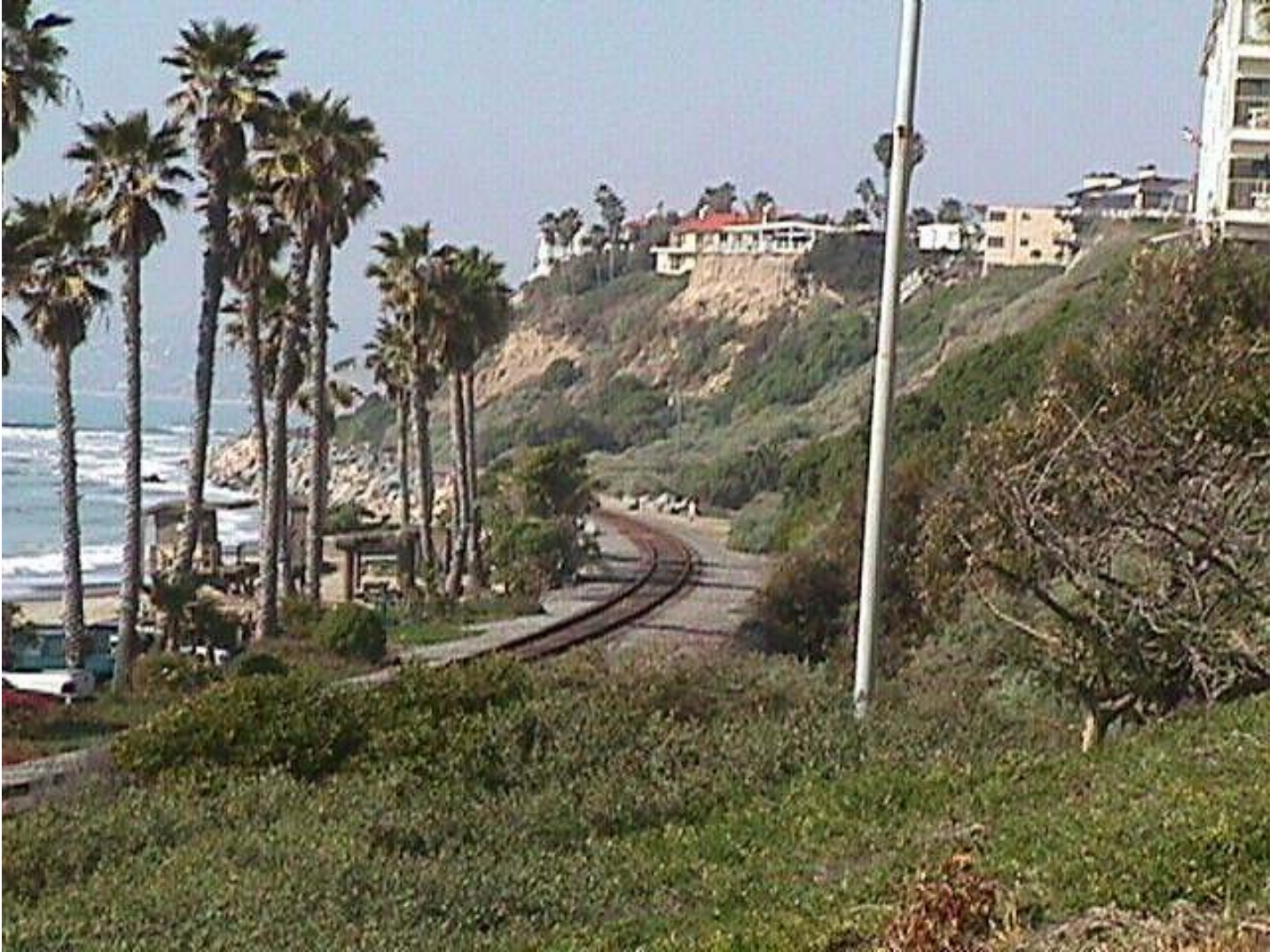
Figure 6-10 – Existing Rail Corridor at Mariposa Point
