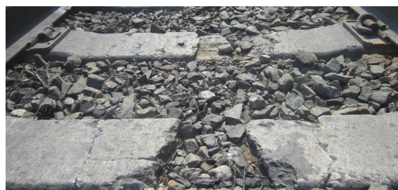
Figure 2. Severely deteriorated crossties in track
