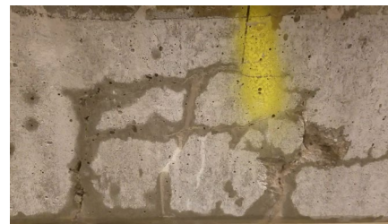
Figure 9. Horizontal cracks along prestress rows
