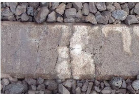
Figure 1. Center-cracked concrete crosstie
