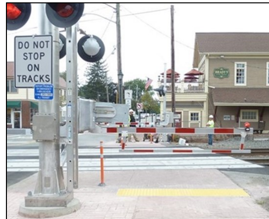
Figure 1. Gate Skirts Installed at E. Main St. Crossing in Ramsey, NJ
