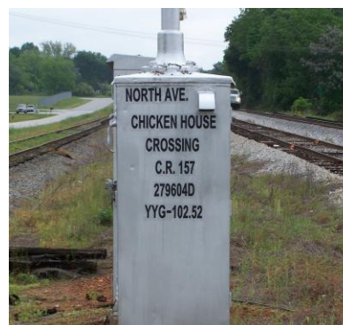
USDOT ID (279604D) on signal equipment enclosure
