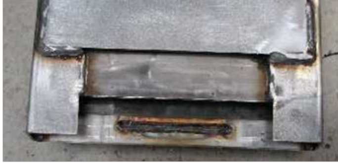
Figure 54. Welded doubler plate
