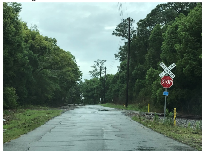
Photo 6: View of Orange Grove Road, at rail crossing, looking west.
