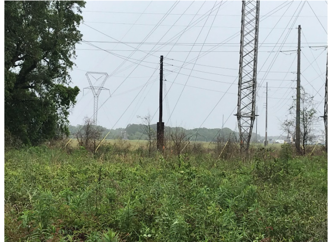
Photo 2: Another View toward marsh portion of proposed North Rail Connector location.
