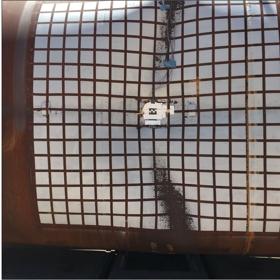
Figure 19. Tank Car After the Impact (impact side)
