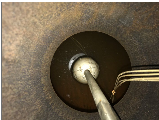
Figure 8. Float installed in tank, looking down through top nozzle
