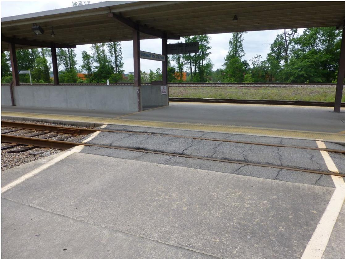
**Figure 6-12. Non-Level-Entry Boarding Island Platform with Vertical Pedestrian Access. Source: USDOT**
