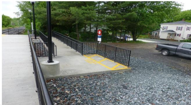
**Figure 3-2. Picture Showing A Ramp Leading from the Backside of a Platform to an Emergency Egress Area; The Landing at the Bottom has an Open Side with an Approximately 9- to 12-Inch Drop Off to a Rocky Surface. A parking lot with a truck parked in it is visible in the picture.**
