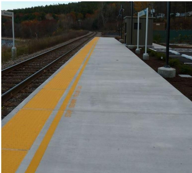
**Figure 7-3. Seasonal Station with a Platform Less Than Full-Train-Length. Source: USDOT**
