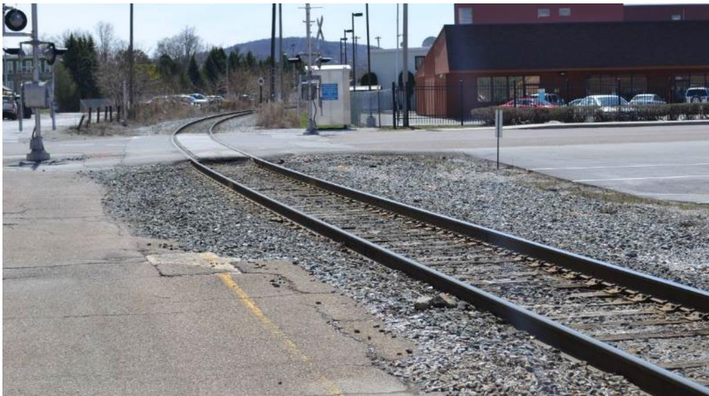
**Figure 4-7. Roadway At-Grade Crossing. Source: USDOT**
