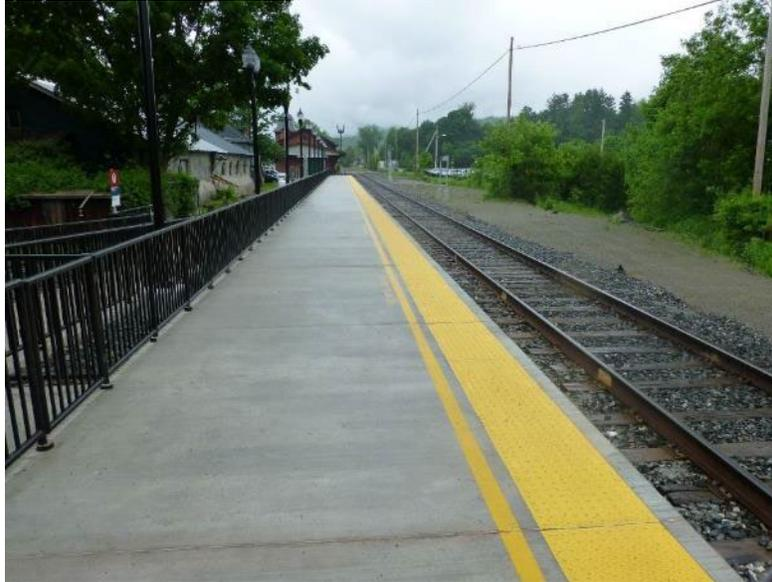
**Figure 4-3. Side Single-Track Railroad Platform Configuration. Source: USDOT**
