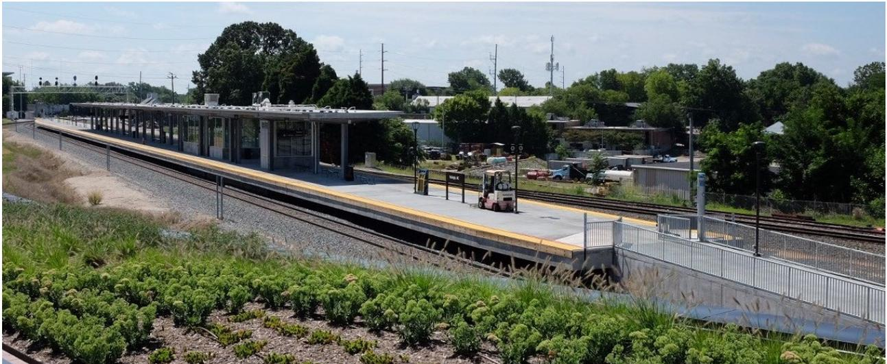
**Figure 6-8. Level-Entry Boarding Island Platform with Vertical Access. Source: USDOT**
