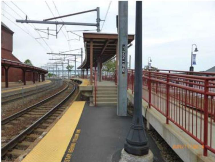
**Figure 5-4. Platform with an 8-Degree Curve. Source: USDOT**
