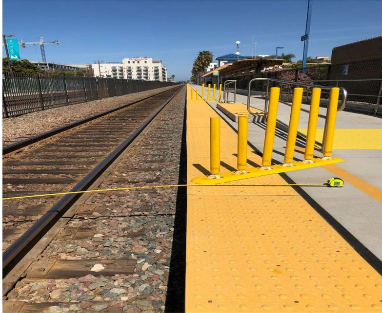
**Figure 3-3. Picture Showing A Mini-High Set Back Platform with ADA-Compliant Edge Protection Preventing the Flow of Pedestrians through the Narrow Area; A Tape Measure Shows Where the Commuter Authority Intended to Start the Protection to Comply with the State’s Public Utility Commission Railroad Clearance Standard. Source: USDOT**
