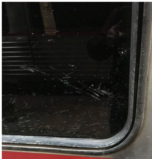
Figure 38. Exterior window with zip-strip removed
