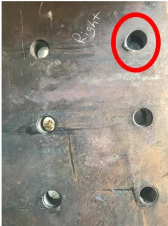
**Figure 53. Deformed Bolt Hole in Draft Pocket**
