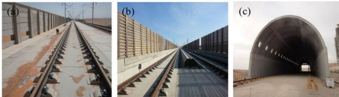
Figure 6-11. Main wind protection structures along the Lanxin Railway II [17]. (a) Subgrade wind barriers; (b) bridge wind barriers; (c) wind-proof tunnels
