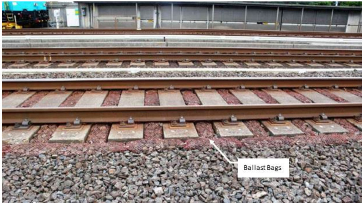
Figure 10-4. Japanese ballast bags (Figure 3.4 from [45])
