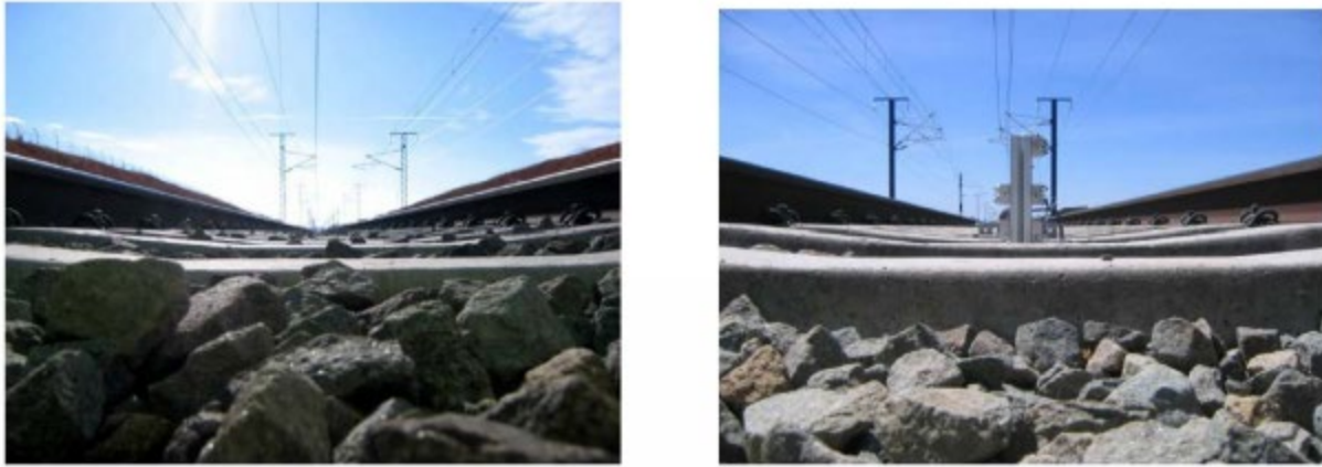
Figure 10-2. Left: Typical track ballast conditions. Right: lowered profile ballast less susceptible to aerodynamic effects from trains (Figure 3.3 from [45])
