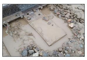
Figure 1. Photograph of mud pumping with standing water
