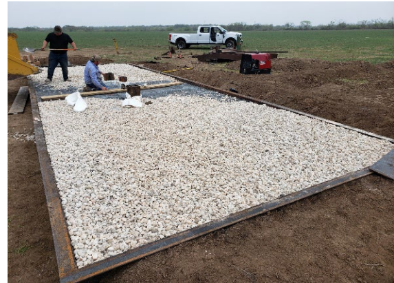
Figure 3. Photograph of LPG Fire Exposure Burner Construction
