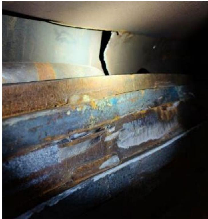
**Figure 104. Right Side of the Cracked Front Plate**
