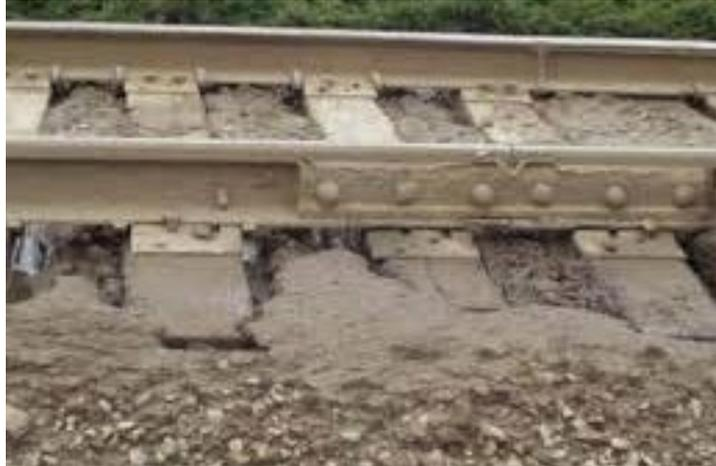
**Figure 2. Example of track segment with fouled ballast**
