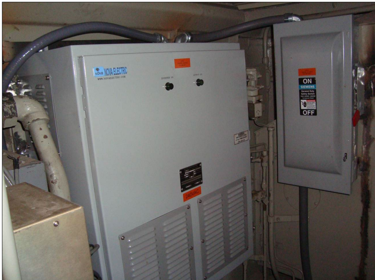
Figure 4. Inverter Inside FRA-2001
