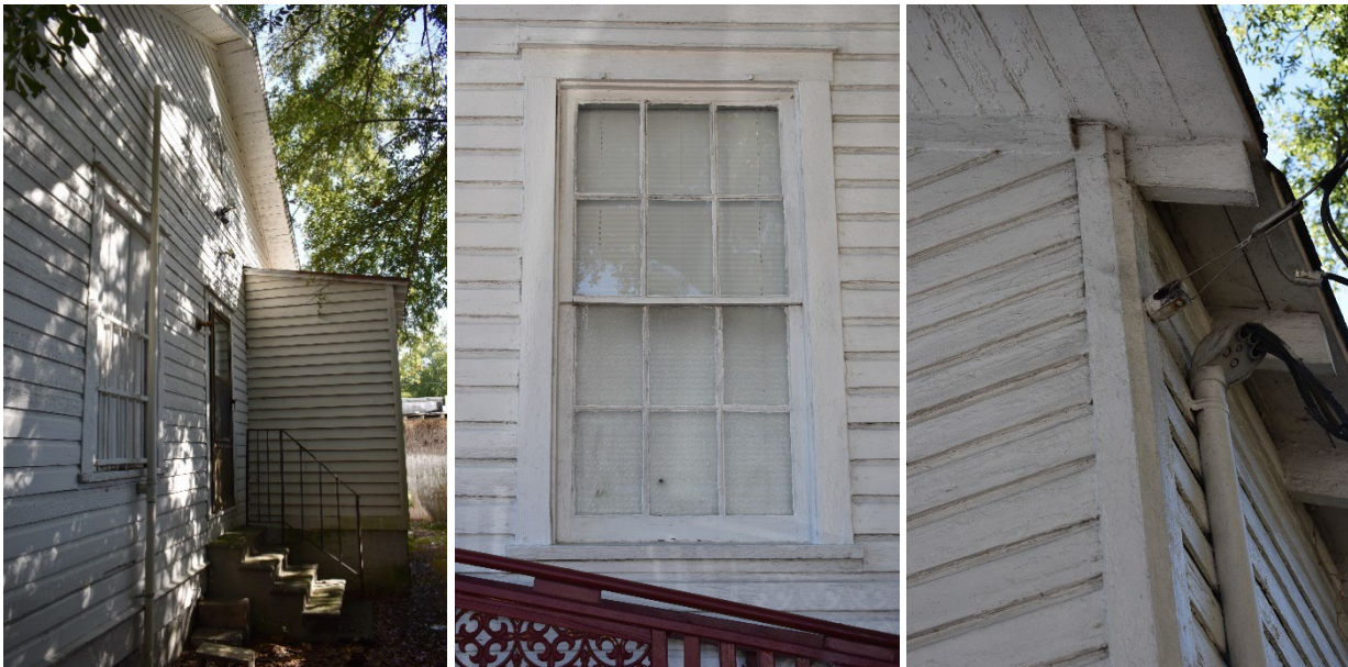
Exhibit 4: Former Holy Church of Jesus Christ, south rear elevation facade, at left; facade window, surround, and ramp railing, at center; German siding and eaves at southwest corner of facade, at right
