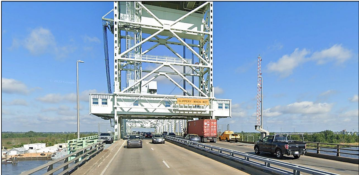
Figure 49: Cape Fear Memorial Bridge—looking west at east tower, lift span, and parking platform framed by green guardrails and holding gate, July 2022 (source: GoogleEarth)
