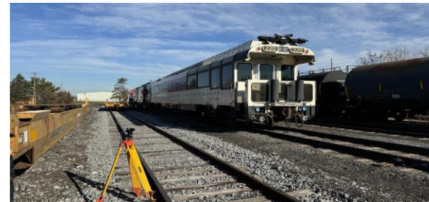
Section of track monitored at Letterkenny, PA
