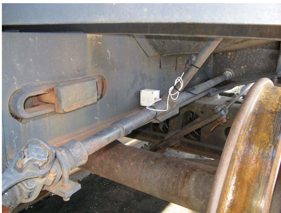
Figure 5. Vertical Accelerometer Mounted on the Stub Sill and Each End of the Car
