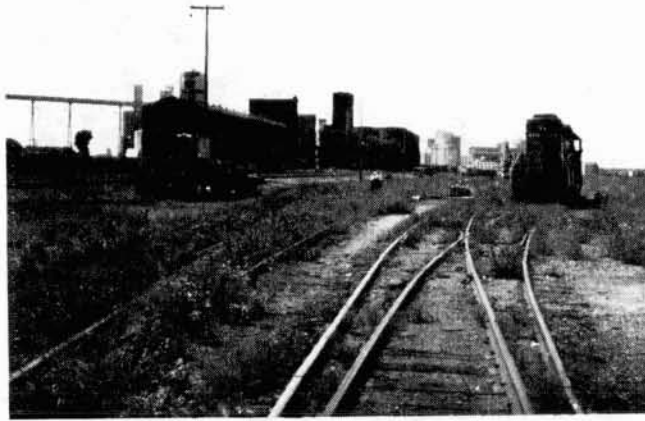
a. View Looking West.
