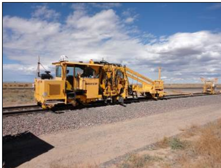
Figure 11. Tamper Used to Complete Surfacing Operations at FAST for this Study
