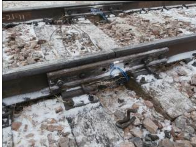
Figure 22. Installation of Instrumented Joints Bars at FAST
