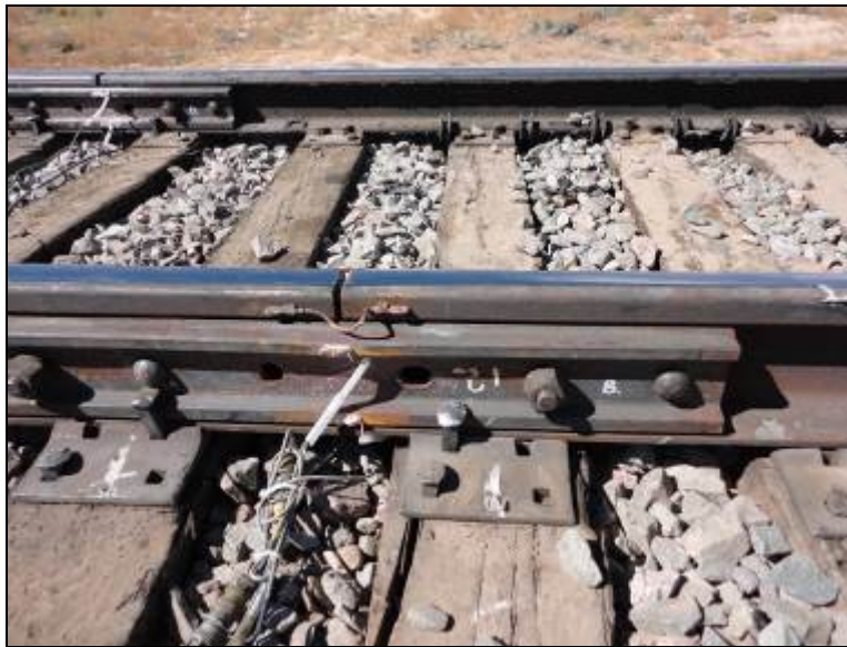
Figure 7. Installation of the Joint Bars in the Test Zone at FAST
