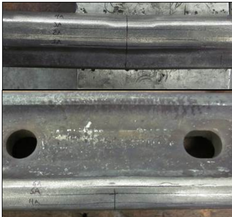
Figure 17. Longitudinal Profile Measurement Locations at the Top of a Test Joint Bar
