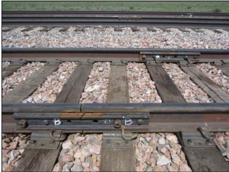
Figure 18. Installation of Standard and Post-Hardened Joint Bars at FAST
