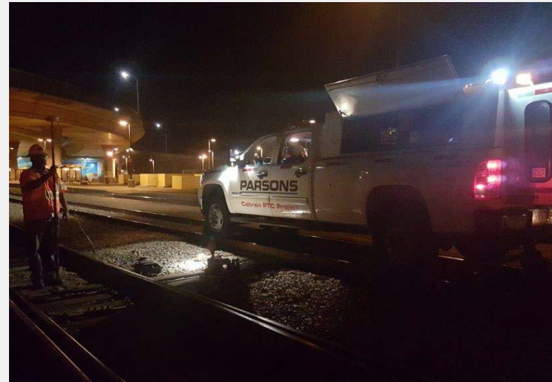
Integrated testing on PTC territory at turnout.
