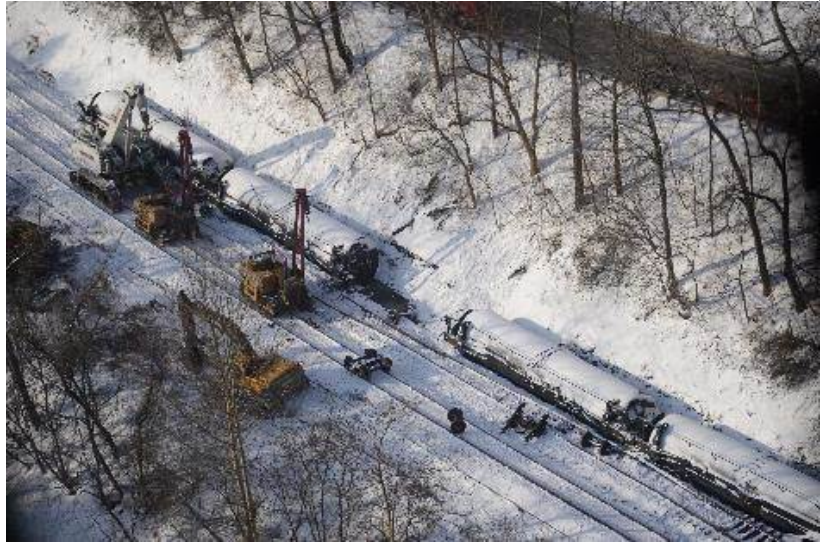
Figure 7: Re-railing tank cars.
