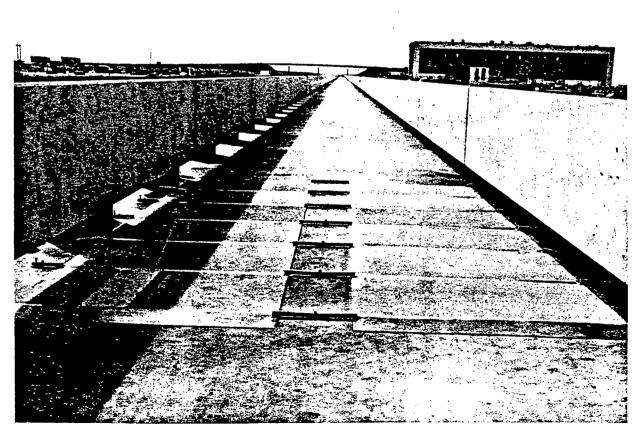
Figure 6. Surface Irregularities in TLRV Guideway to Study Vehicle Response and Behavior.
