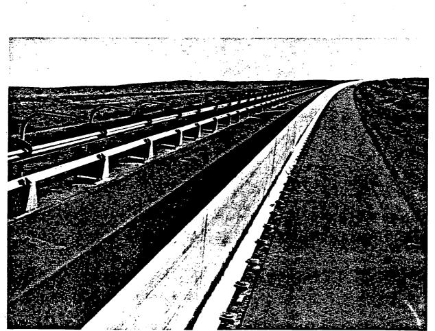
Figure 8. PTACV Guideway at Transportation Test Center. Reaction Rail in Center and Power Distribution Rails on Left.
