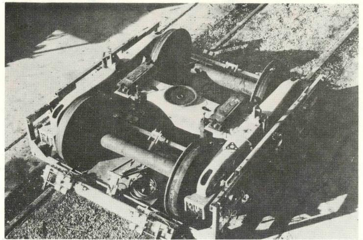
Figure 3-9. Air Bag Side Bearings
