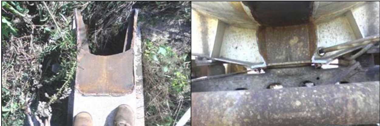
Figure 3. Stub Sill Fracture Observed in Callahan, FL (December 2009)
