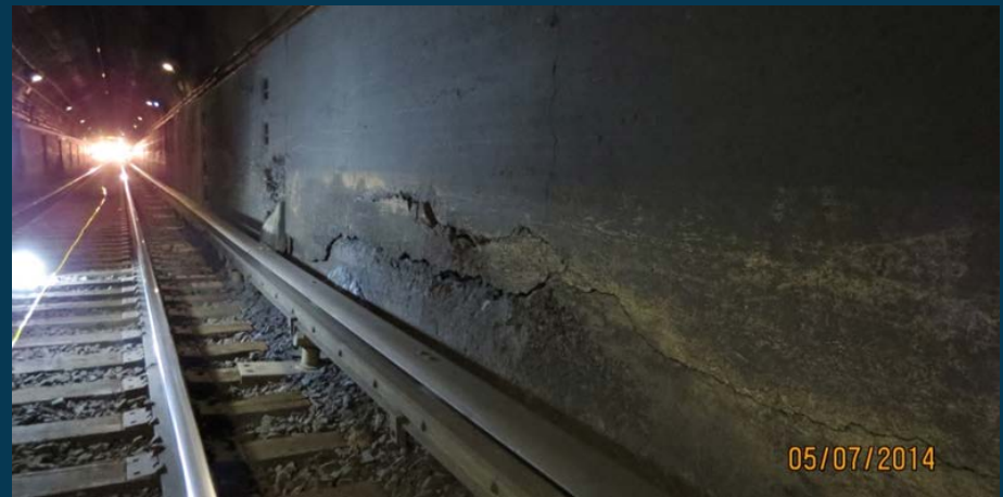
SPALLING OF CONCRETE TUNNEL LINER
