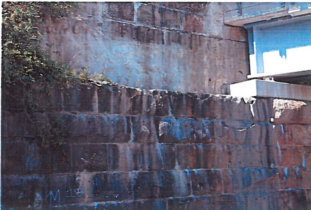
Patching & leaching at Adams Street
