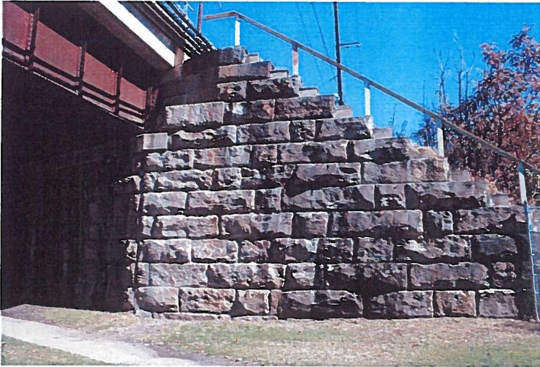
Chop-down & capping at Stokes Street abutment
