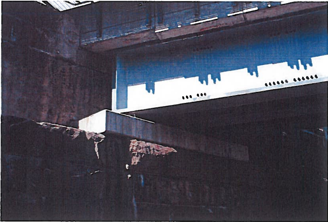
Concrete capping & chop-out at Adams Street
