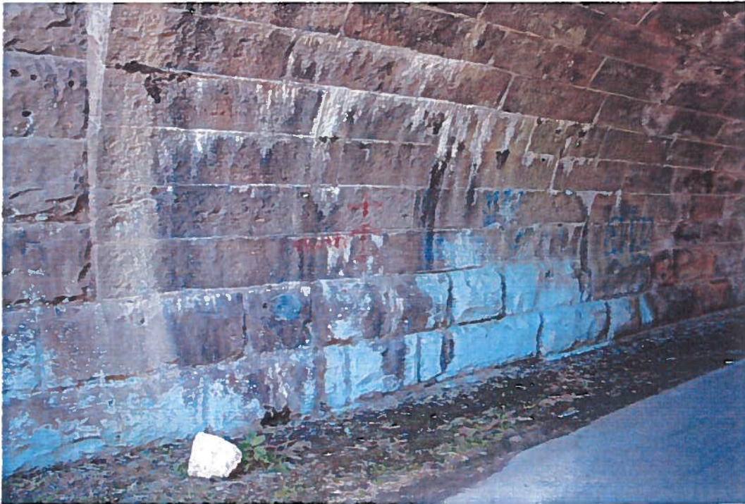
Leaching & discoloration within Centennial overpass
