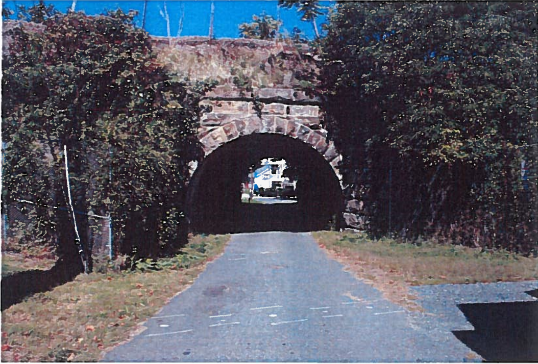
Freedom Lane overpass, south end
