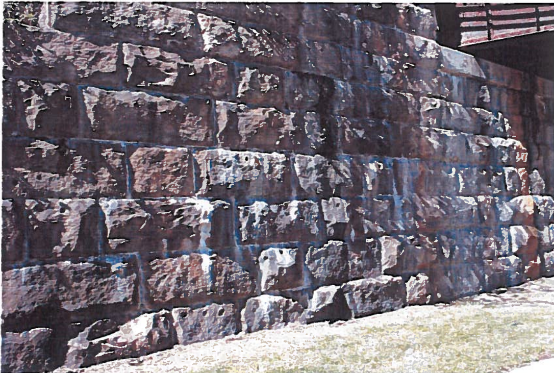
Leaching & leaking at Stokes Street abutment
