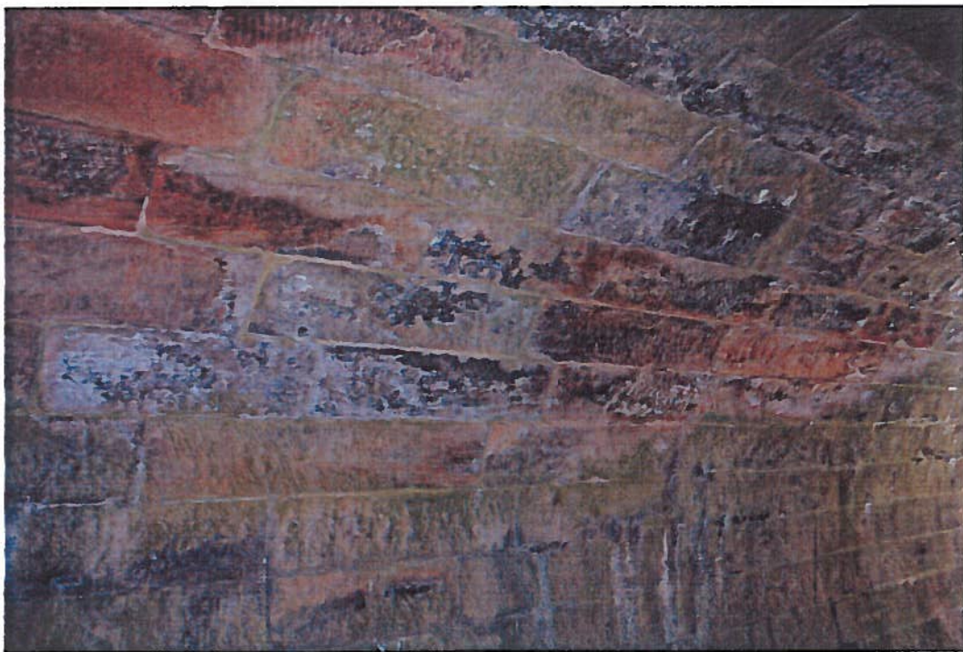
Leaching & discoloration within Freedom overpass
