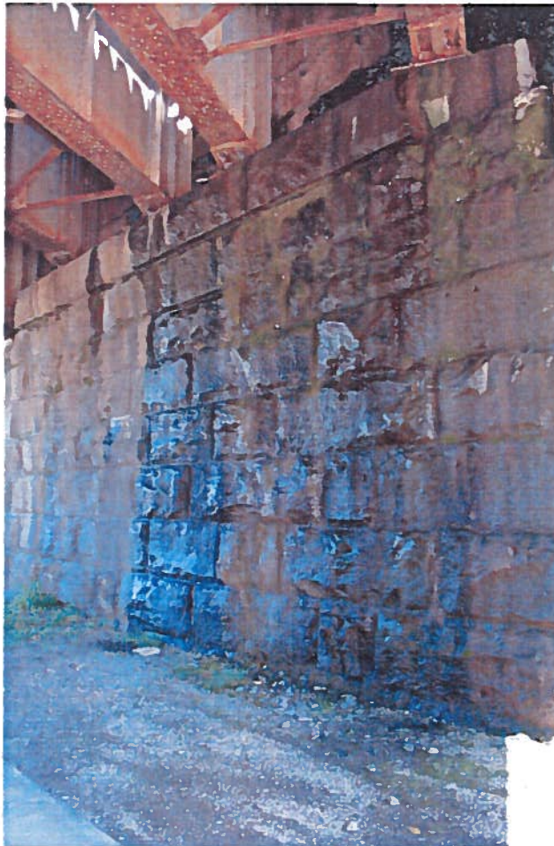
Abutment leakage, deterioration & discoloration at Juniata Street
