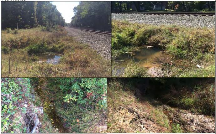
Top Left: View of clogged culvert under railroad Top Right: View of clogged culvert under railroad Bottom Left: Typical view downstream Bottom Right: Typical view downstream
