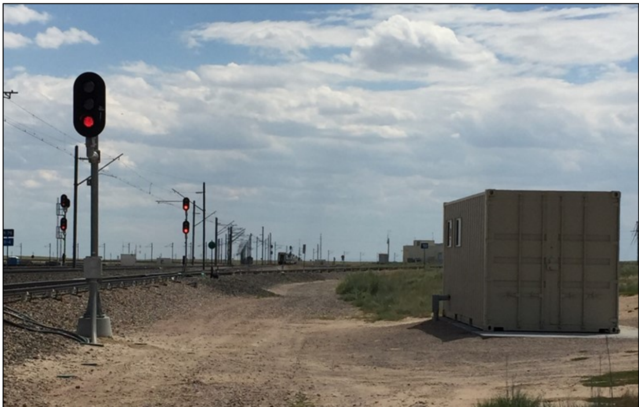
Figure 10. Signal Stand Installation at T51.7 (Control Point)
