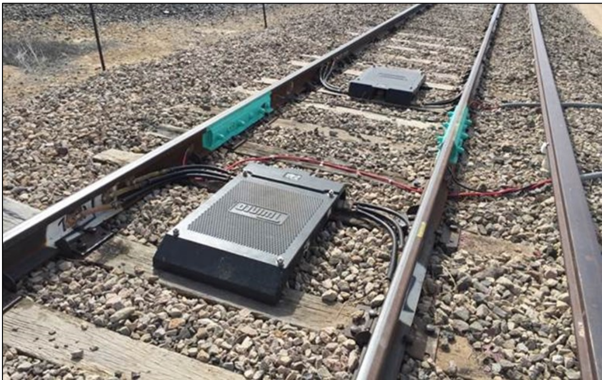
Figure 9. Installation of Insulated Joints and Impedance Bonds
