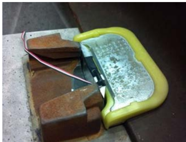
Figure 26. LLED Installation Prior to Clip Application
