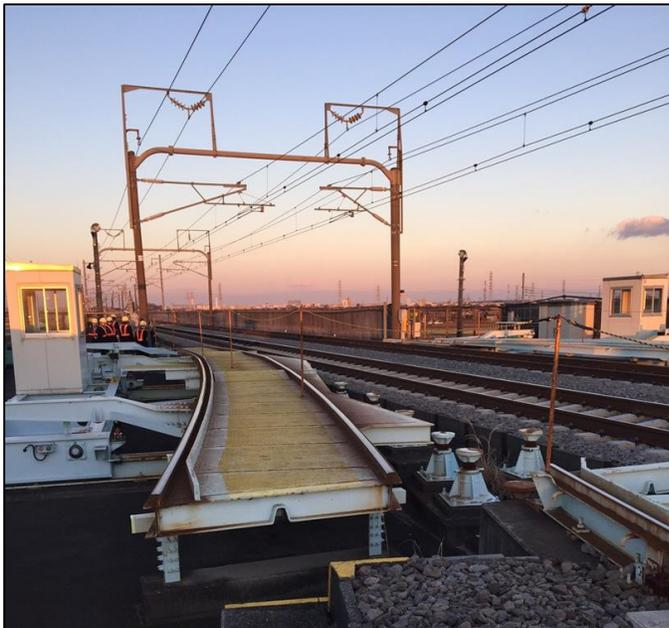
Figure 33: Mechanical Siding-off Temporary Track Connection
