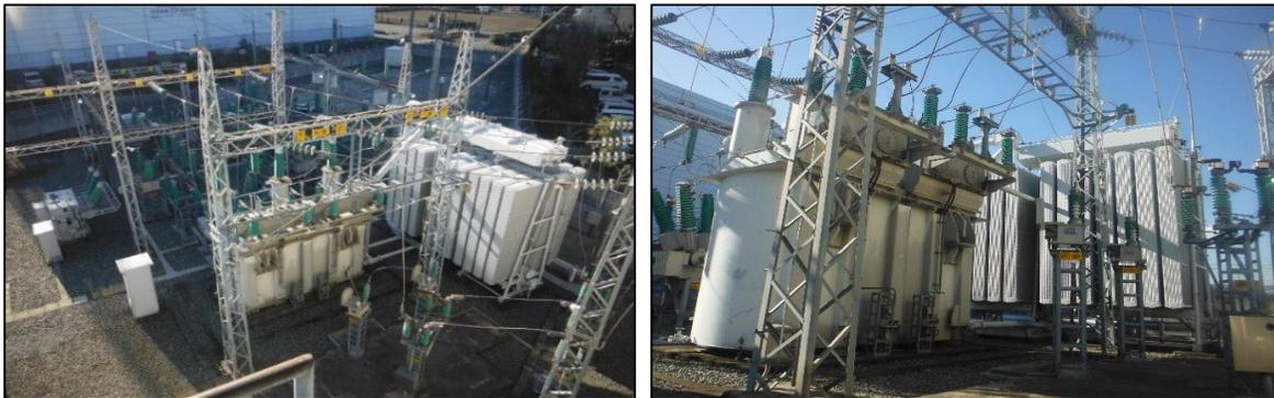
Figure 17: Typical Traction Power Transformers
