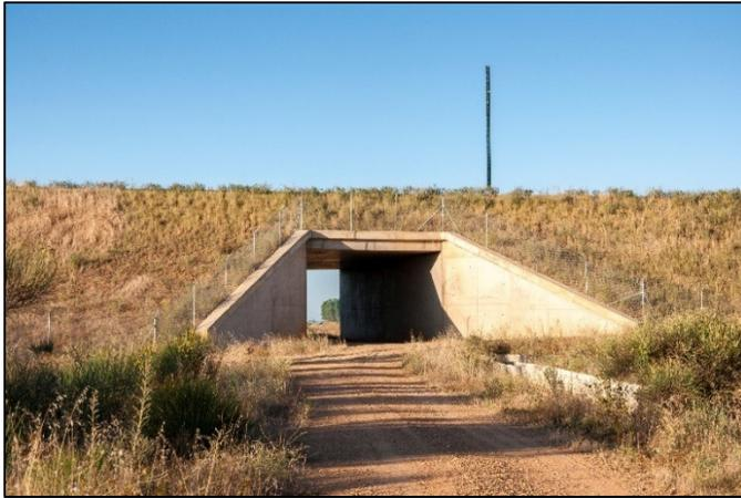
Figure 43: Example of a multifunctional wildlife crossing in a road embankment. Note clear line of sight, vegetated entrance, and large opening to accommodate cattle and wildlife.
