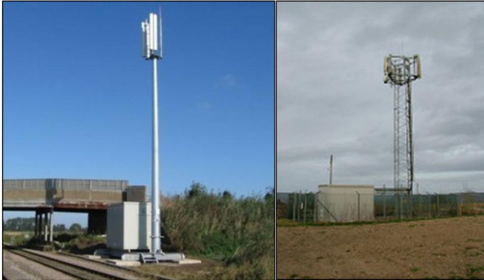
Figure 30: Typical Monopole and Lattice Mast and Antenna at Grade
