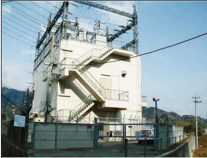
Figure 25: Typical Building of Sectioning Post (SP), Sub-Sectioning Post (SSP), Auto Transformer Post (ATP)
