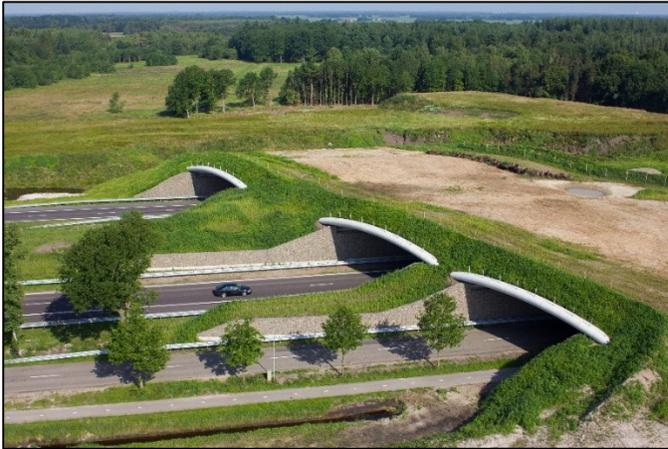
Figure 42: Example of recently constructed wildlife highway overpass crossing.
