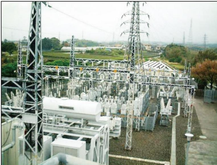
Figure 18: Photo of Typical Traction Power Substation on Tokaido Shinkansen in Rural Area
