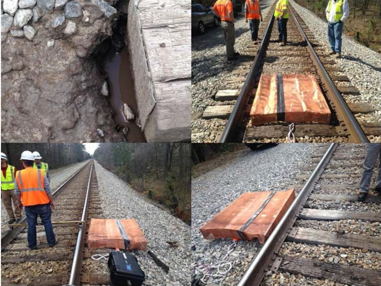
**Figure 21: Milepost 68.3, close-up of mud-fouled ballast and photos of three measurement locations.**
