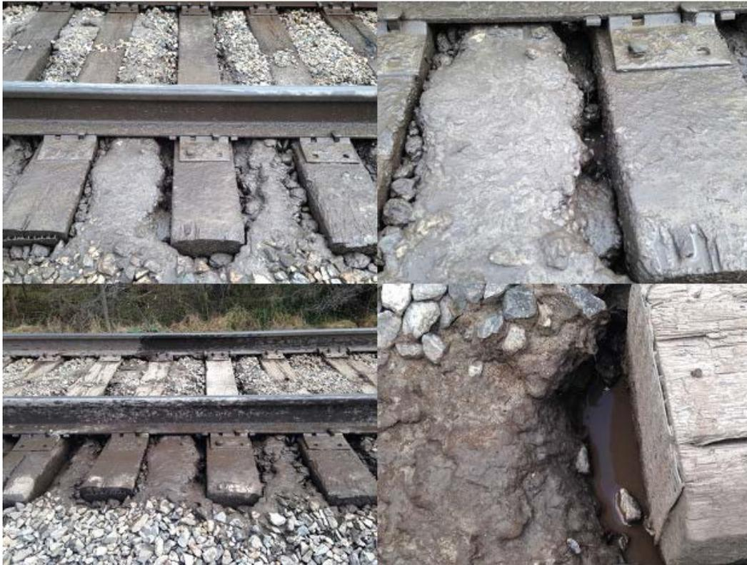
**Figure 14: Close-up photos of some of the mudholes over which TMMS measurements were performed.**
