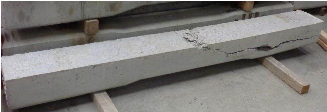
A Sample of a Broken Through Concrete Tie
