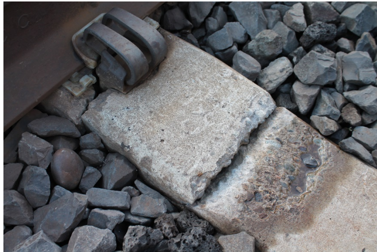
Crosstie Transversely Broken Between the Rail Seats
