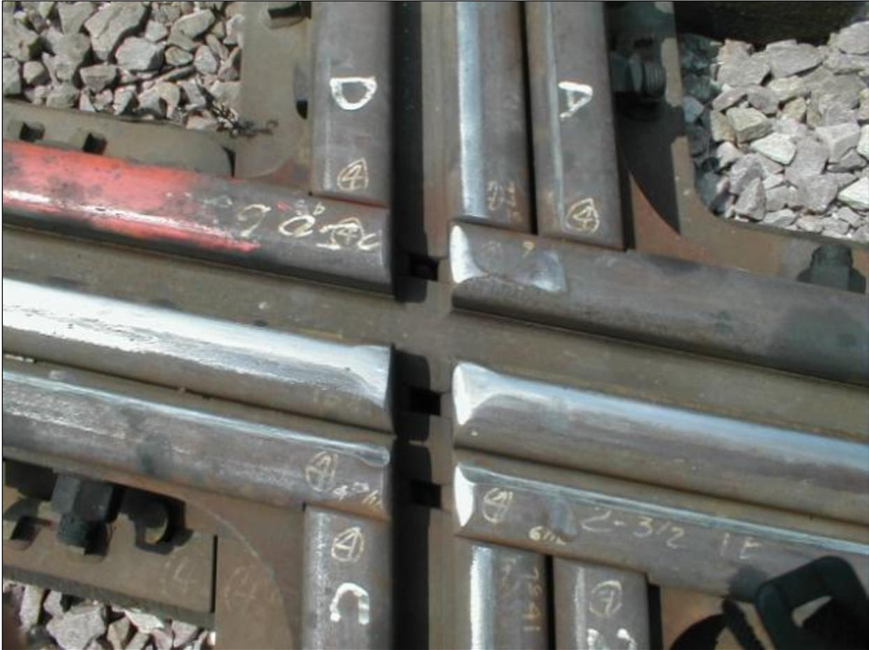
**Figure 3. Three-Rail Crossing in Revenue Service**
