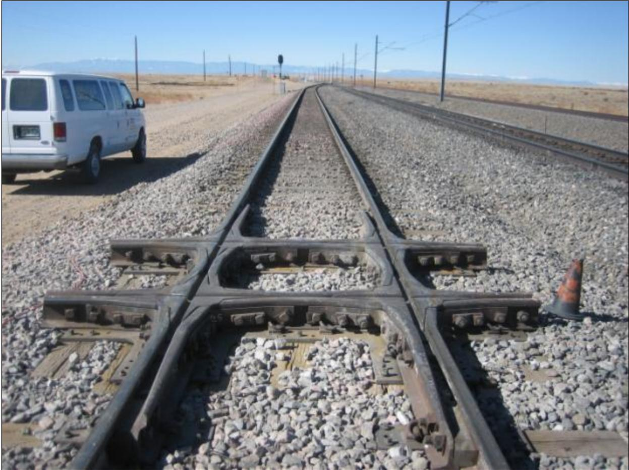
**Figure 2. Cast Diamond Crossing Tested at FAST**
