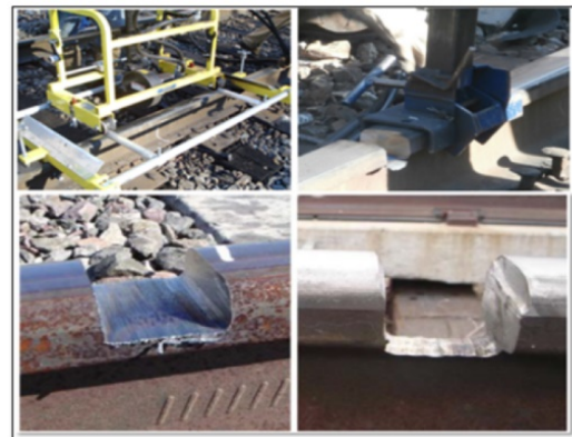
Figure 2. Supplier A's Process Requires a 1-Inch Slot (left) and Supplier B's Process Requires the Slot to be the Depth of the Full Railhead (right) (Gutscher, D., 2009).
