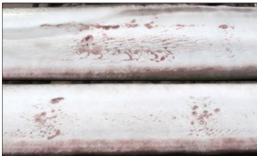
Figure 3. Head-Defect Repair Weld Installed on the Low Rail: Supplier A (top) Supplier B (bottom).
