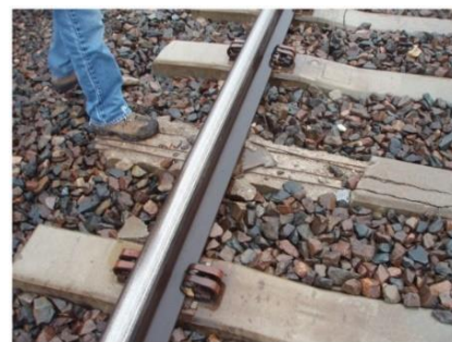
Figure 1 : In-Track Crosstie Failure
