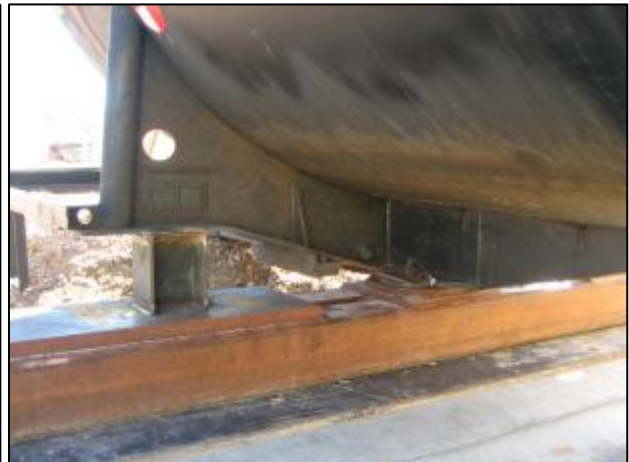
(b) Welded I-beam connection
