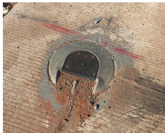
Figure 13 – Example of dirt accumulating on in-pavement light fixture
