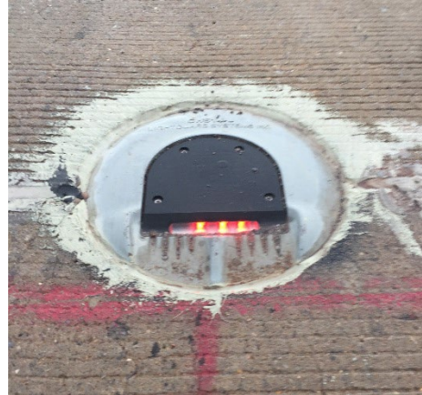
Figure 14 – Light with Burned out LEDs
