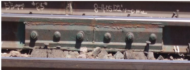
Figure F-3. Bonded Insulated Joint
