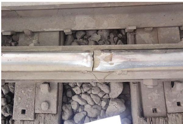
c) Deteriorated and Battered Down Rail Ends
