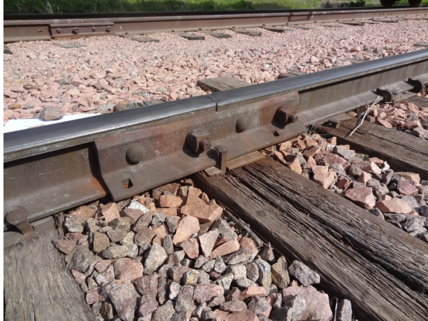
a) Field Side View of an Intact Joint
