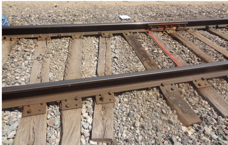
b) Skewed Ties and Fouled Ballast
