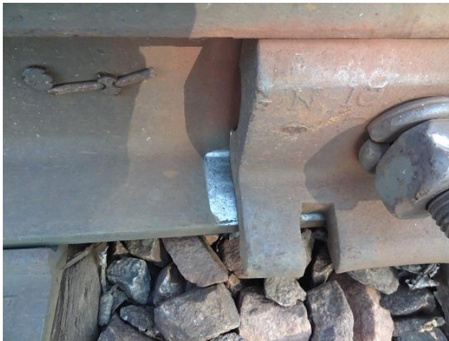
b) Detail of Scratch Mark on Rail Base
