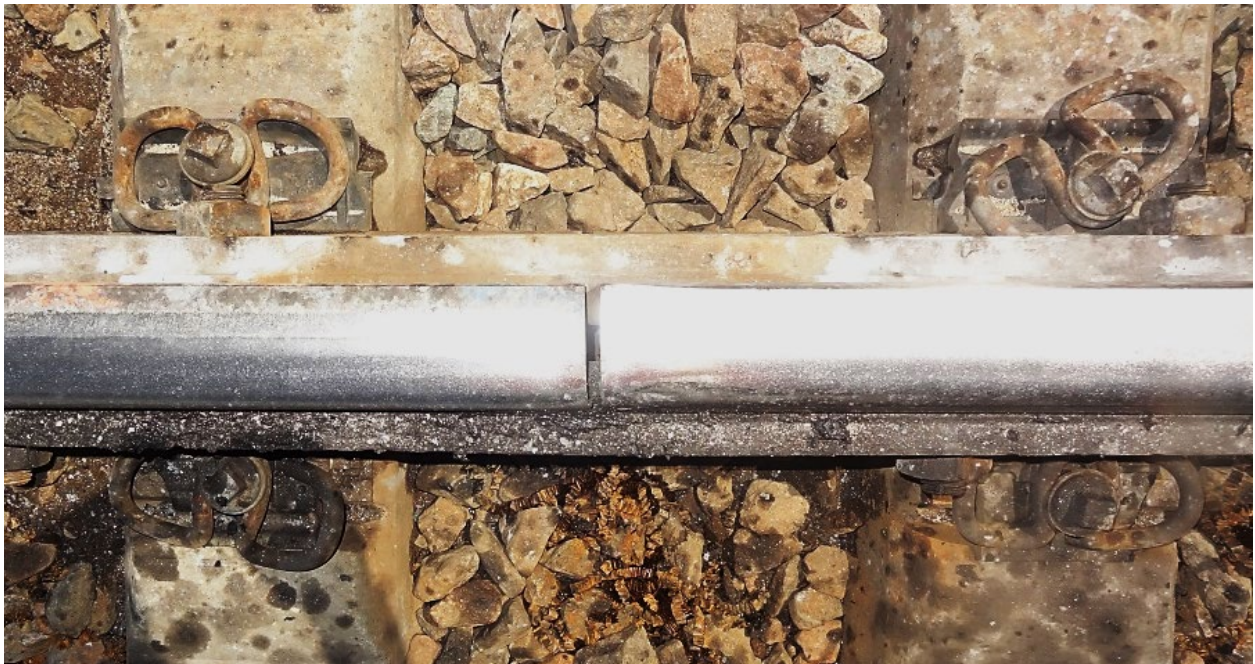
Figure 20. Temporary Joint on Concrete Ties Fully Equipped with VOSSLOH Fasteners
