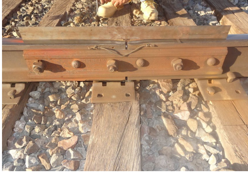
a) Rail End Batter at Location #120726-001-0404
