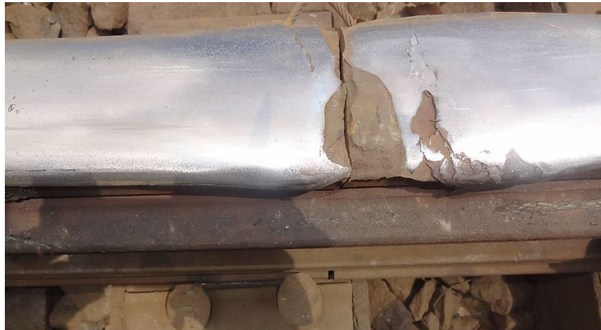
b) Deteriorated and Battered Down Rail Ends
