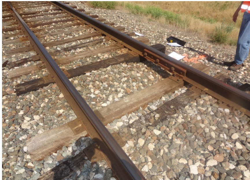
b) 40'' Tie Spacing at Location #120723-010-0232
