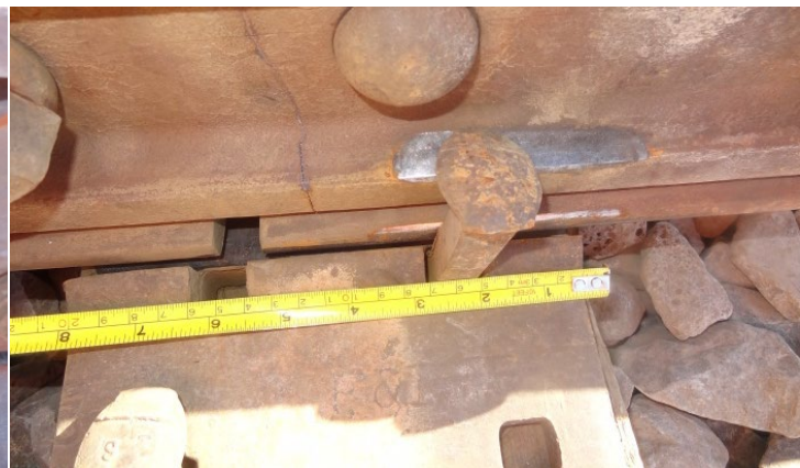
e) Sign Longitudinal Movement near a Fastener
