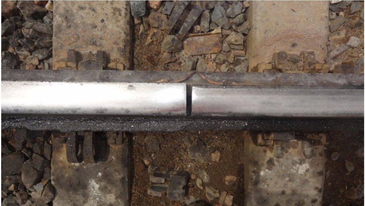
Figure 19. Temporary Joint on Concrete Ties Not Configured with Two Fasteners on the Same Rail
