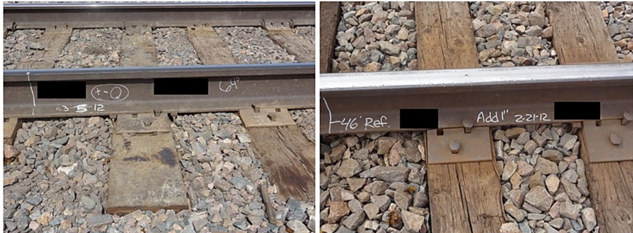
Figure 18. Examples of Welder Reference Marks at Temporary Joints on Wooden CWR Track
