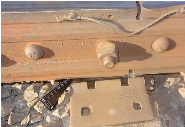
b) Measurement of Gap between Rail Base and Tie Plate
