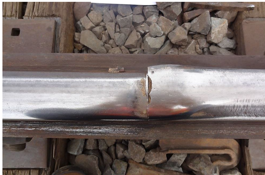
b) Battered Down Rail Head
