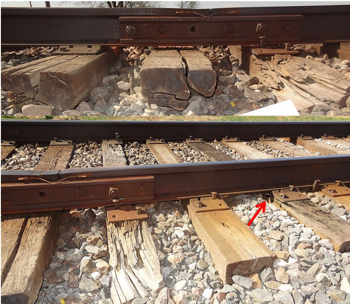
Figure 8. Large Vertical Movement and Wide Deflection Basin at a Failed Rail Joint Location
