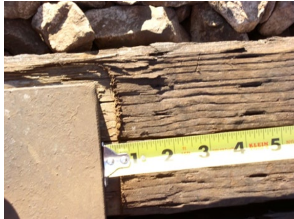
Figure F-11. Evidence of Tie Plate Movement
