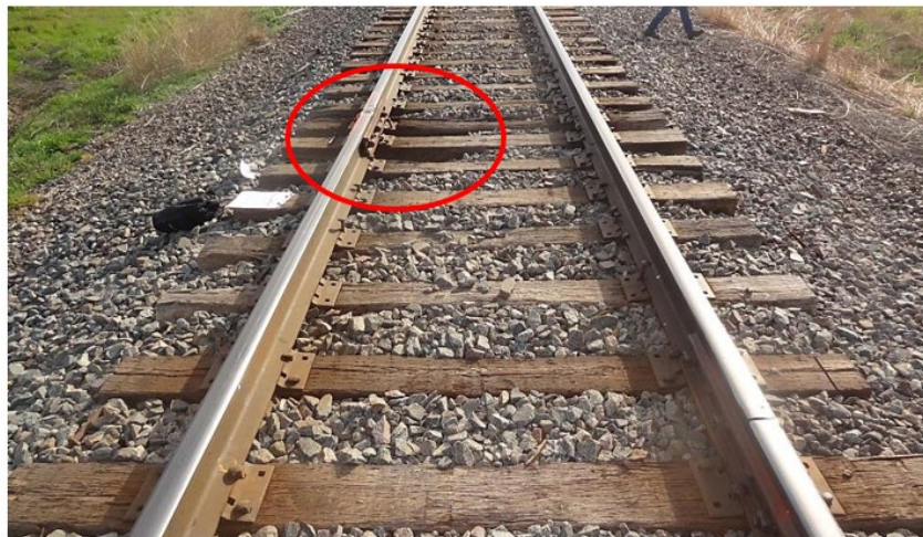
b) Insufficient Ballast at Rail Joint
