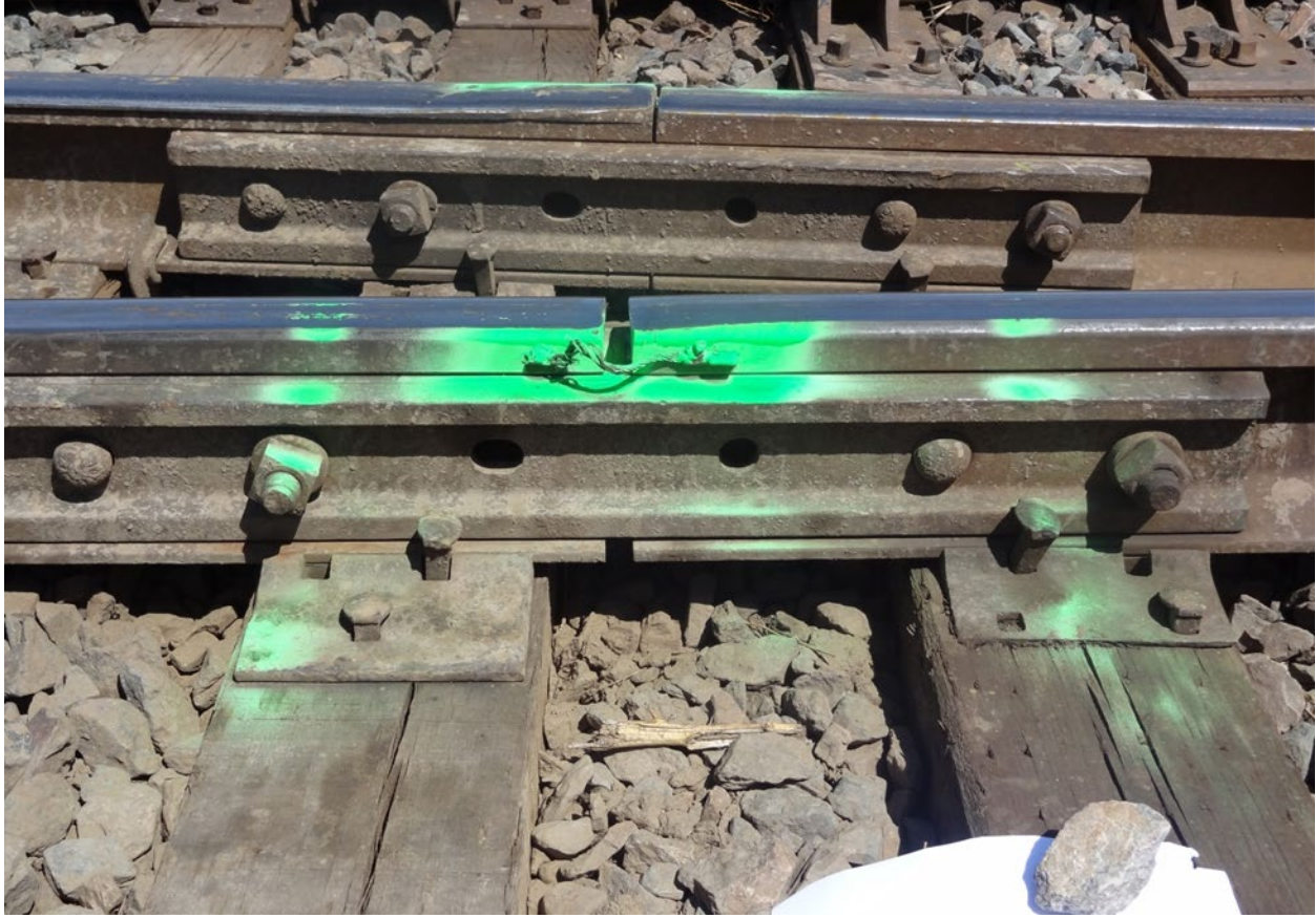
Figure 15. Failed Rail Joint at CWR Territory at Location of Recent Track Work
