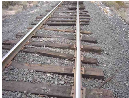
Figure F-10. Results of Lack of Rail Anchors
