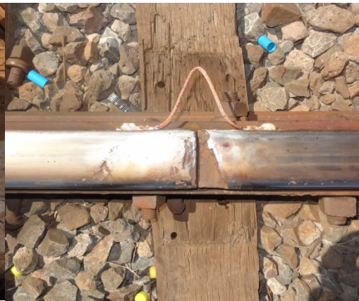
d) Chipped Rail Ends
