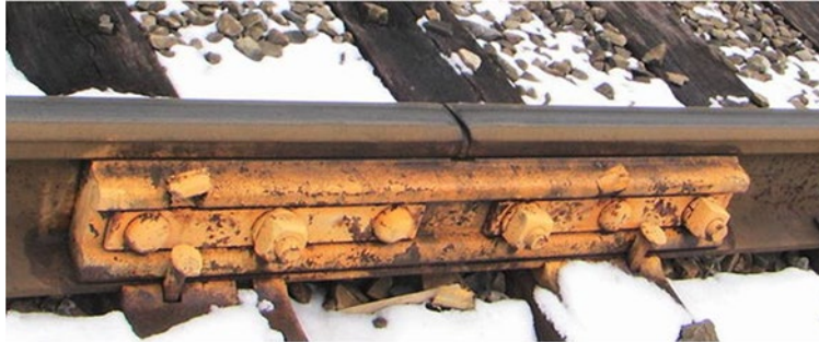
Figure F-2. Insulated Joint with Insulation Material Coating Bar
