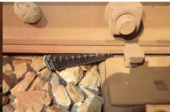
d) Gap between Rail and Tie Plate
