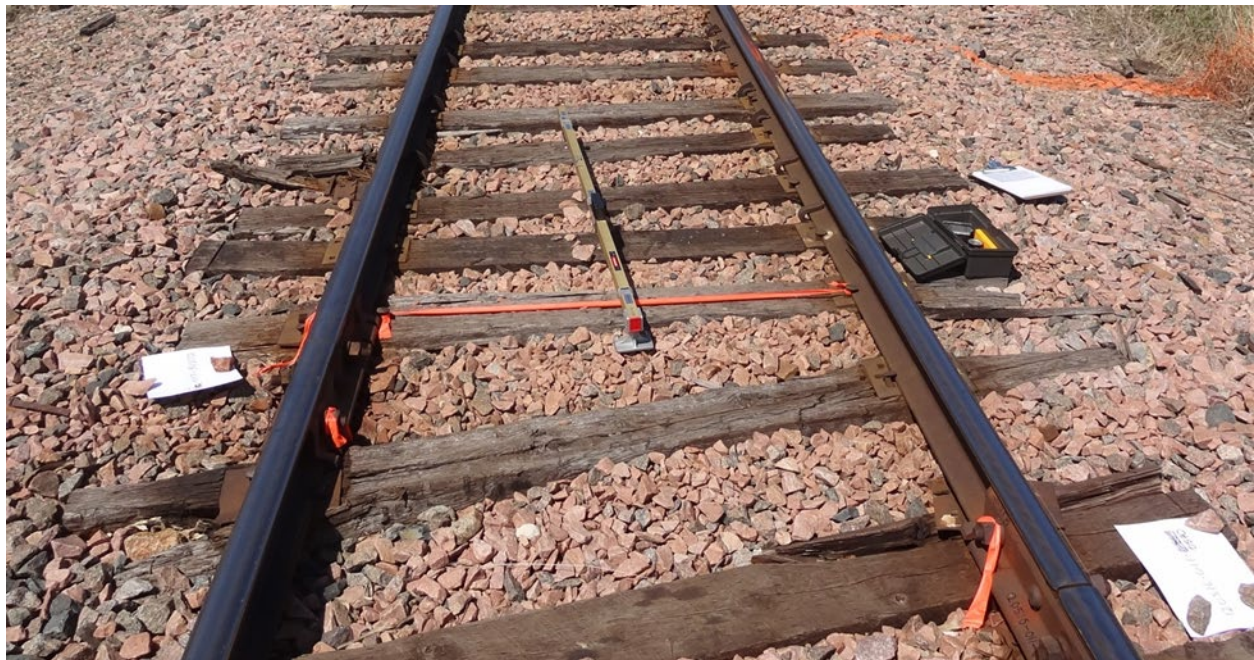
Figure 12. Large Rail Longitudinal Movement and Skewed Ties
