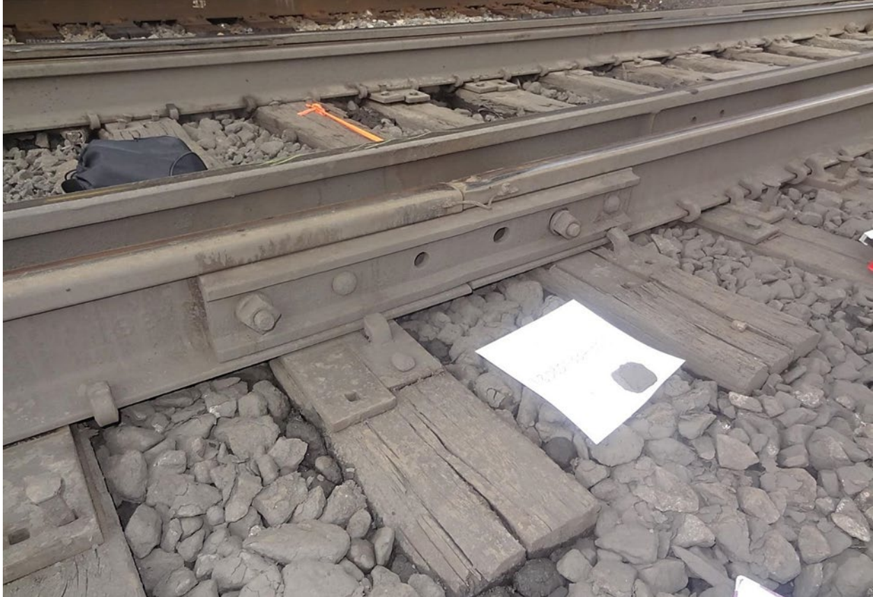
Figure 14. Failed Rail Joint at CWR Territory with Deteriorated Support and Rail End Conditions
