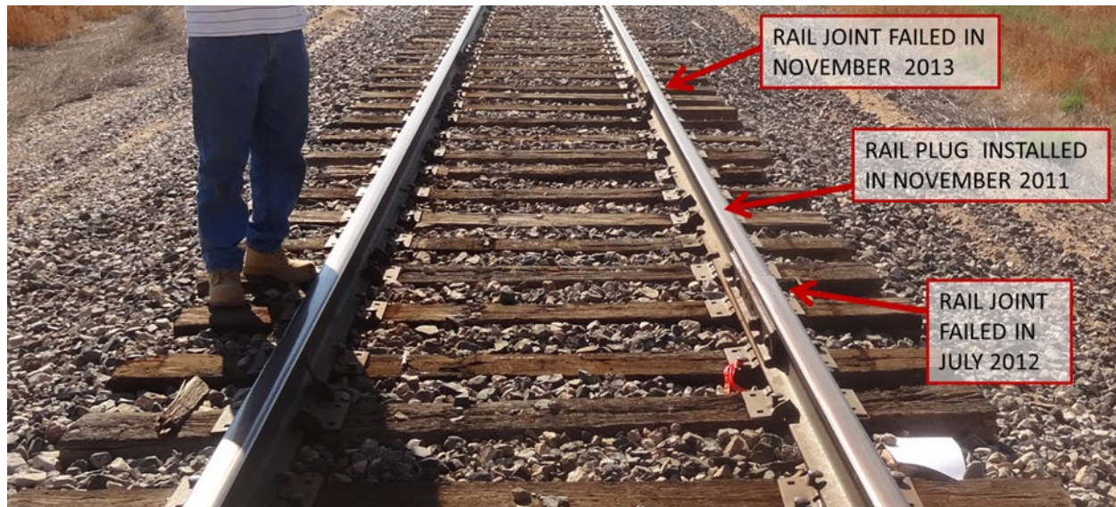
Figure 76. General Field Conditions in the Vicinity of a Recently Installed Rail Plug
