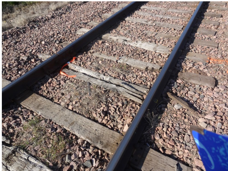
b) Fouled Ballast in a Vicinity of a Failed Joint
