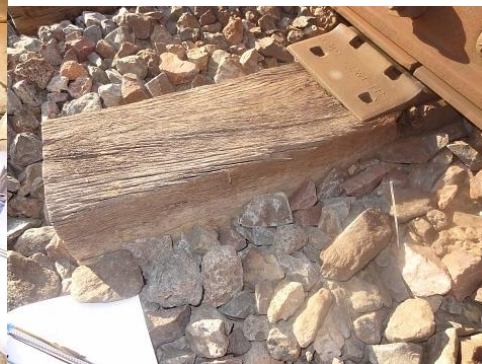
d) Signs of Tie Pumping on the Side of the Tie
