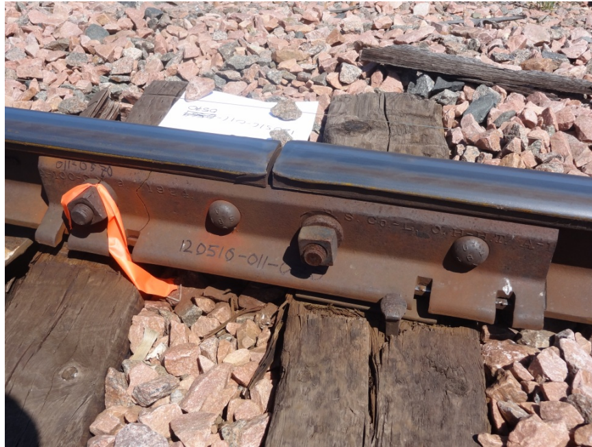
a) Gage Side View of a Rail Joint Defect in the Area of Large Longitudinal Movement
