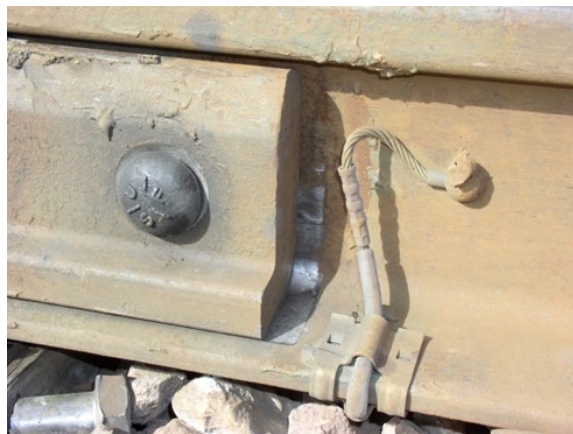
Figure F-9. Illustration of Evidence of Longitudinal Bar Movement
