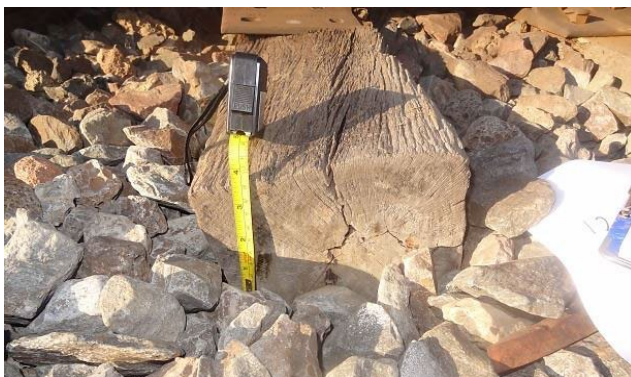
c) Signs of Tie Pumping on the Face of the Tie
