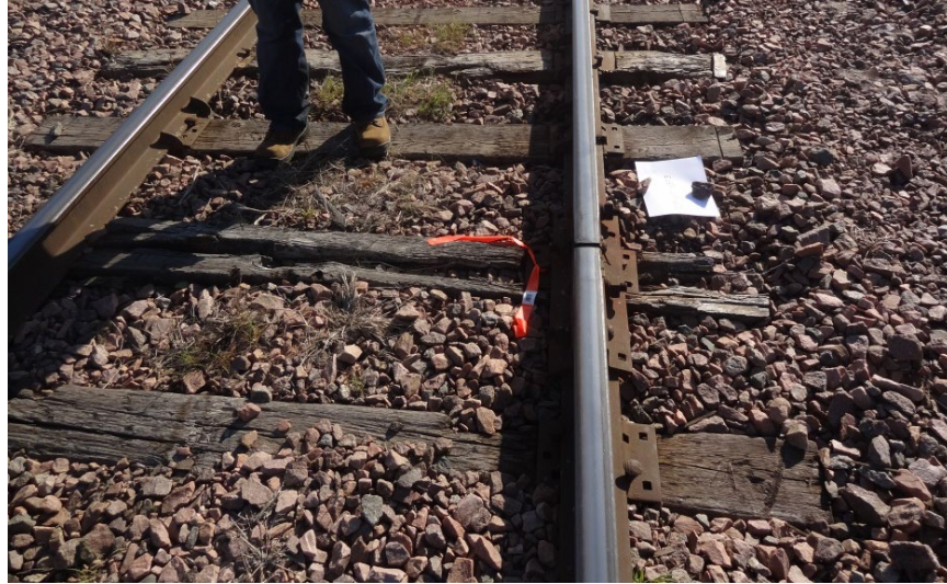
a) Broken Tie under a Failed Joint
