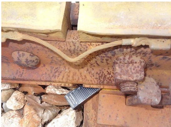
c) Gap between Rail and Tie Plate
