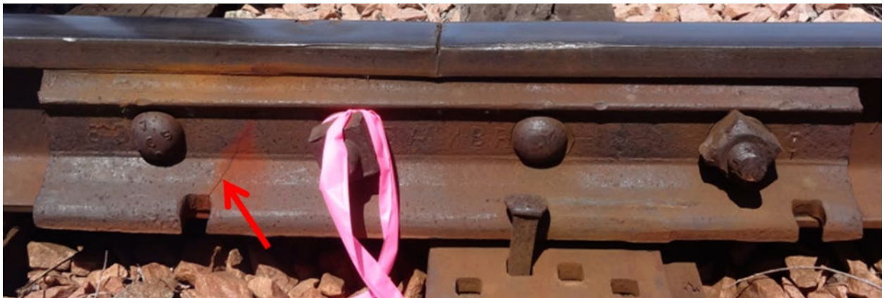
Figure 4. Bottom Quarter Crack on a Long Toe (Angle) Bar Originating at the Corner of the Spike Hole
