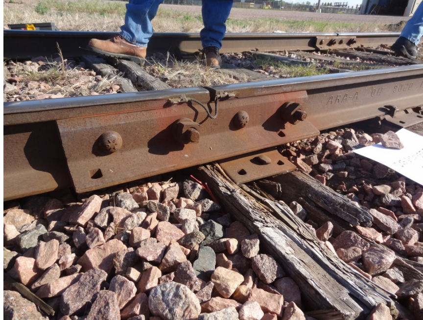
a) Field Side View of a Defect in with Large Longitudinal Movement and Ineffective Tie
