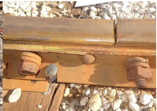
c) Spike in Bar Slot Causing Tie Split
