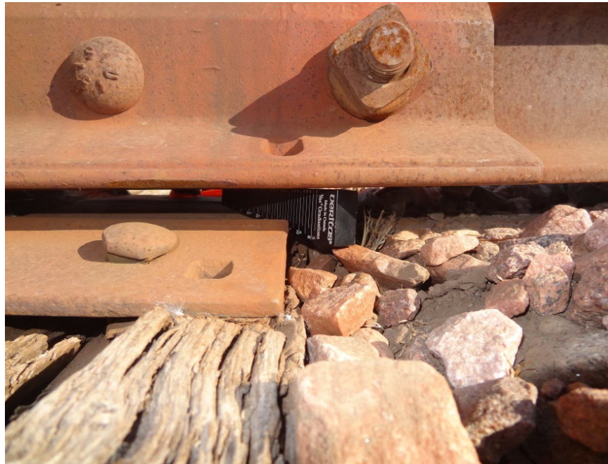
b) Detail of Gap between Rail Base and Tie Plate
