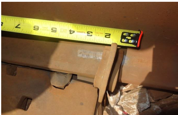
c) Signs of Longitudinal Movement
