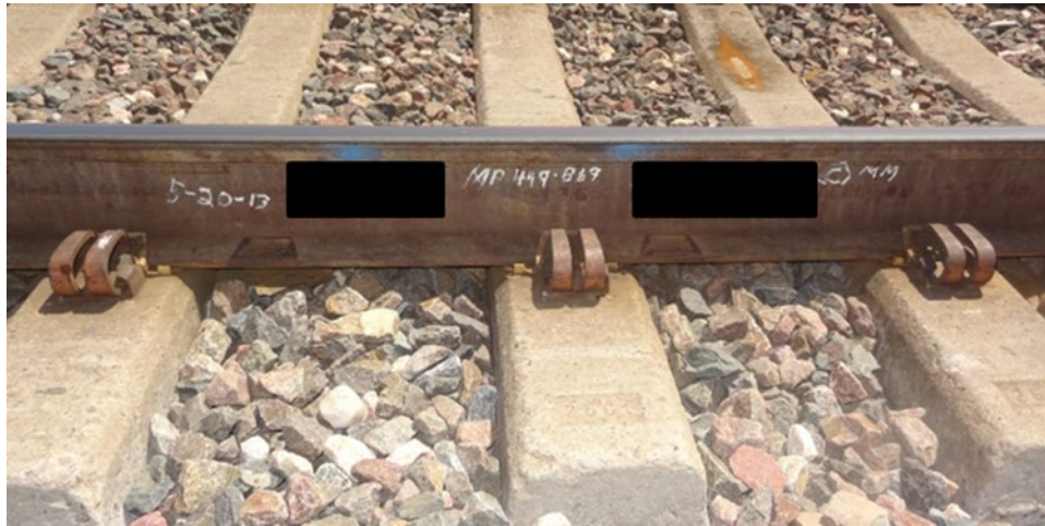
Figure 21. Example of Welder Reference Marks at Temporary Joint on Concrete Tie CWR Track
