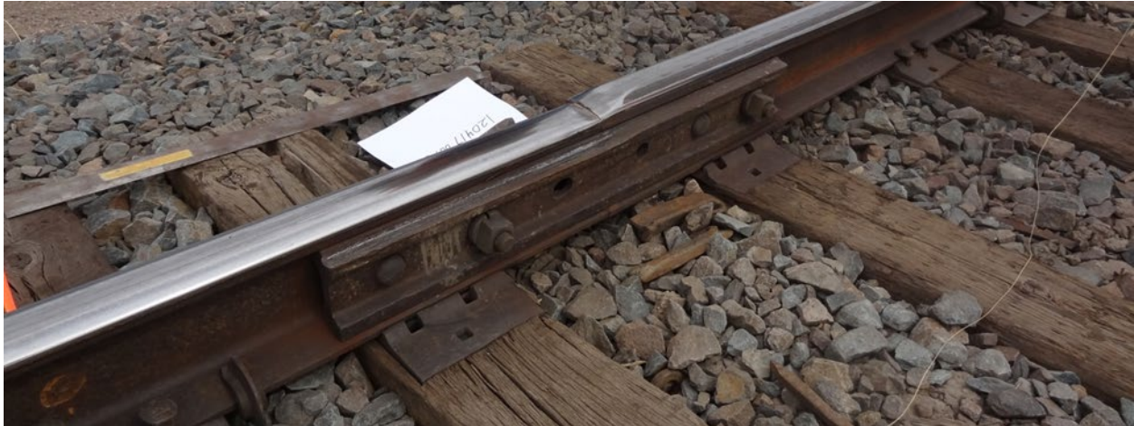
Figure 16. Initially Misaligned Rail End Battered Down into Abrupt Rail End Ramp
