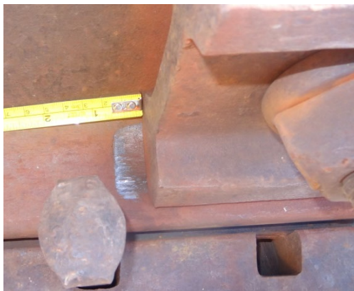
d) Sign of Longitudinal Movement
