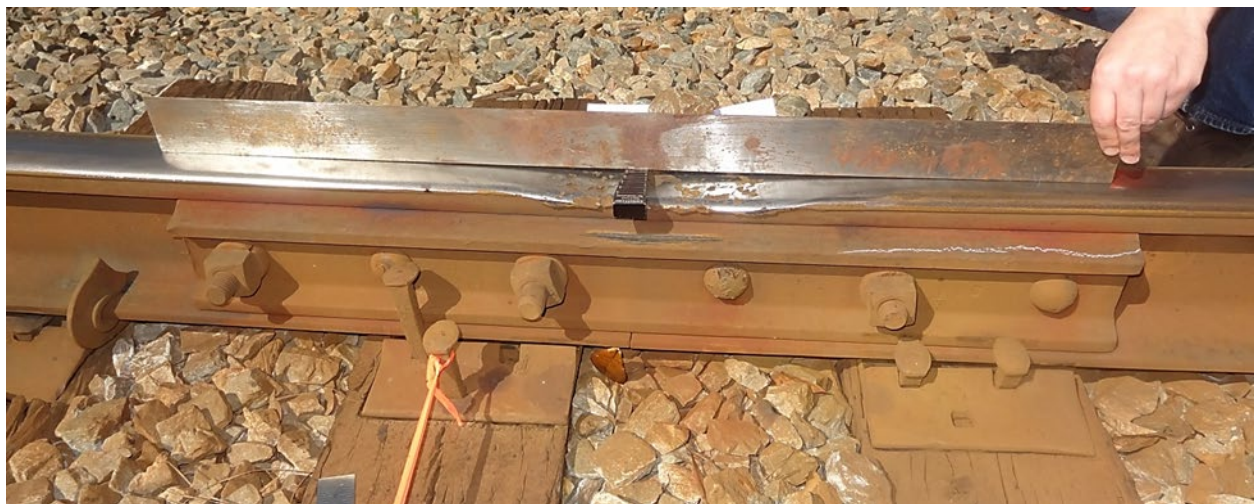
Figure 10. Large Rail End Batter at a Failed Rail Joint Location with Straight Edge to Demonstrate Magnitude
