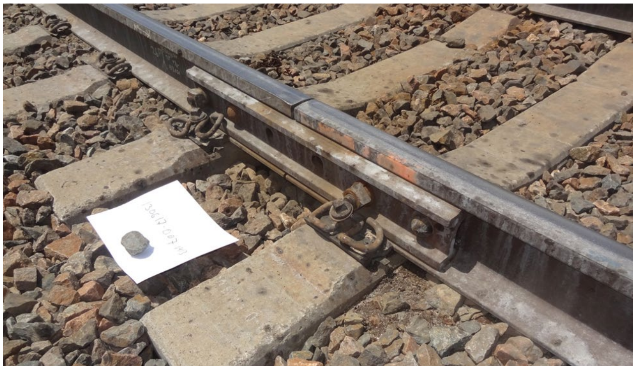
Figure 22. Example of Rail Joint Location on Concrete Tie Track with Good Support Conditions
