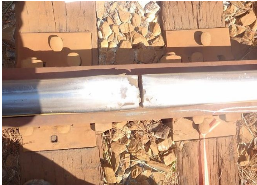
b) Chipped Rail Ends
