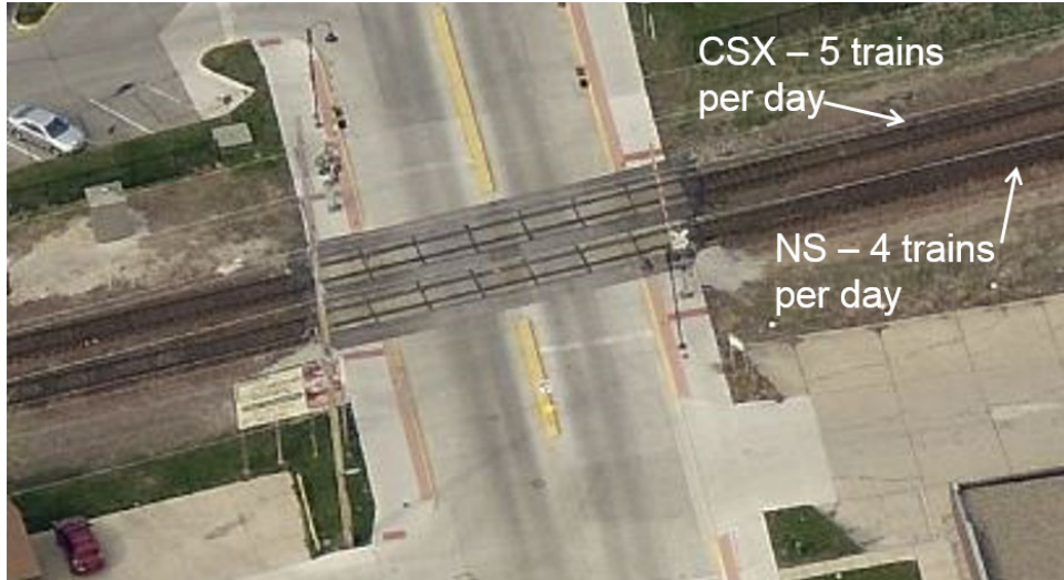
Figure 5: Example of multiple railroads operating on separate tracks at a crossing
